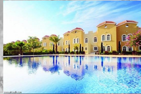
AlQumrah (Phase I) 50 villas
